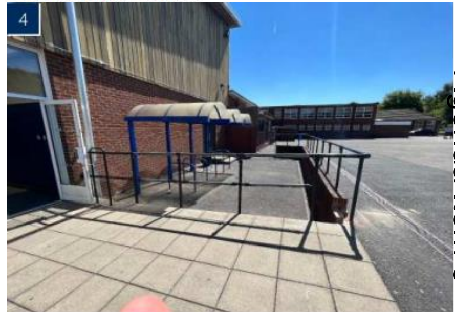
4 Block EFAB entrance from playground/hardstanding, looking south
