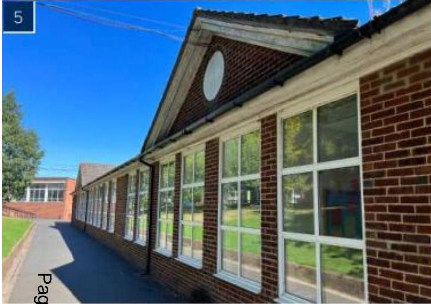
Block of AA west side of quadrangle, looking northwest
